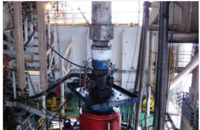
HOLD RCD installed above annular BOP
