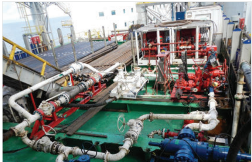
DAPC system installed at cantilever deck
