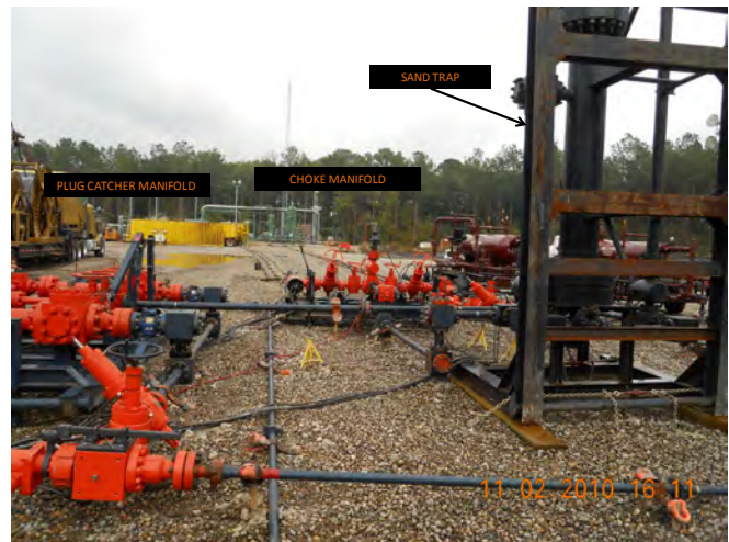
General layout of job showing sand separator and choke manifold.
