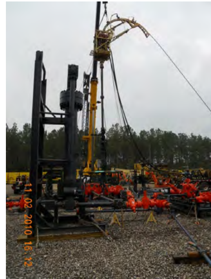
General layout of job showing gooseneck, sand separator and choke manifold
