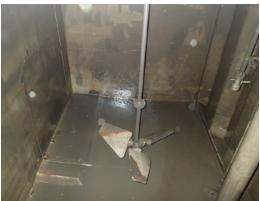
The ATC unit was rigged up using a temporary setup requiring minimum modification or installation to the rig. The 18 pits were cleaned in 61 h 45 min (average time per pit of 3 h 50 min). The pontoon tank was cleaned in 12 h 40 min rather than days using only 44 bbl [7 m³] of washwater. The final total volume was 135 bbl [21 m³] for all 18 pits and the 2,800-bbl [445-m³] pontoon tank. A total of 52.1 tonUK of barite solids was removed.
