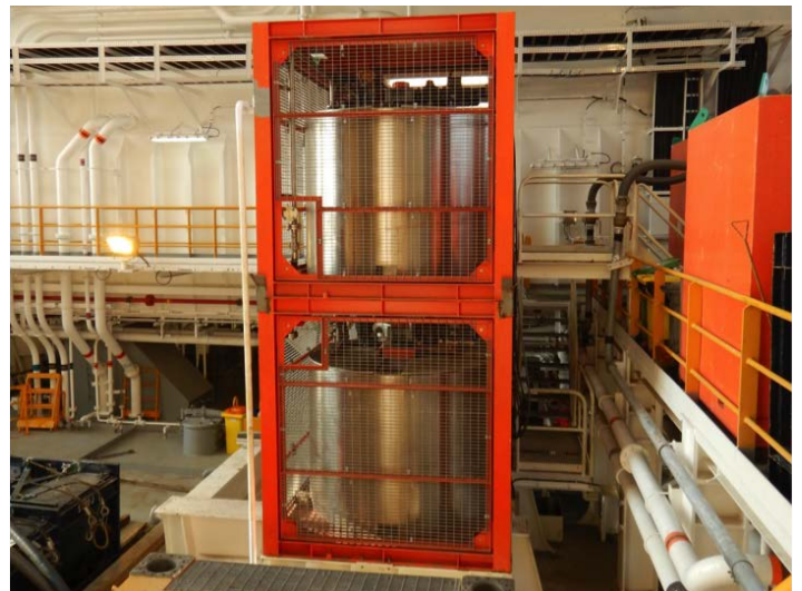
The system provided overall improvement in the QHSE program, helping to reduce transfer of contaminated fluid and decreasing the need for crane lifts of skips and confined space entry for tank cleaning.
